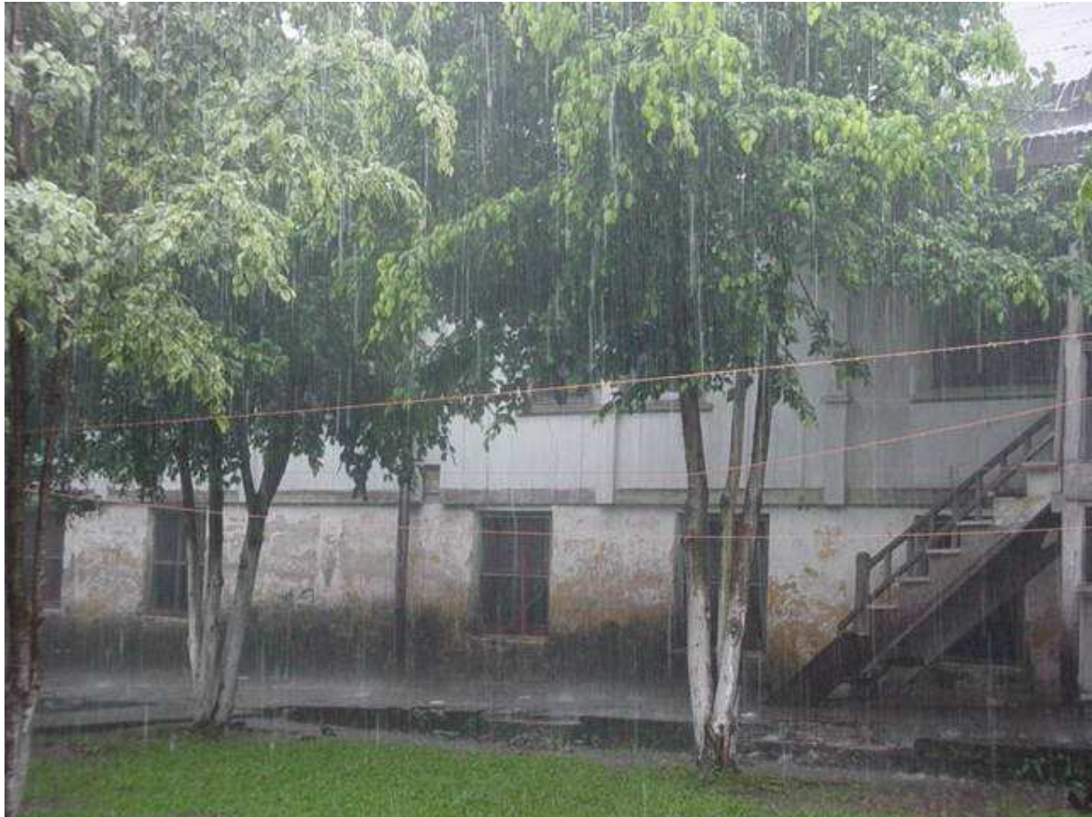
Fig. 1-5. Heavy rain falling on Chocolá , and the old general headquarters area of the Finca Chocolá.
